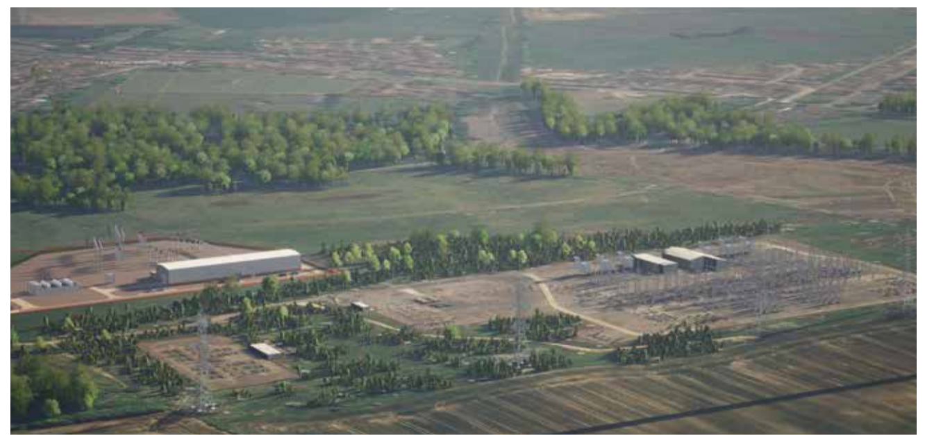
An indicative image of our proposed new substation (in the orange box), next to existing infrastructure.
