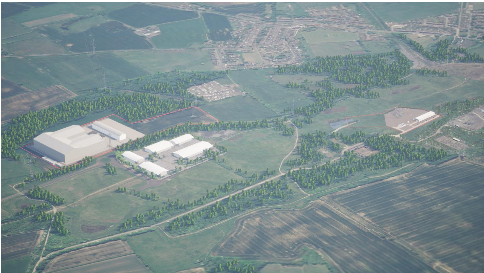
An indicative image of our Hawthorn Pit converter station and substation
